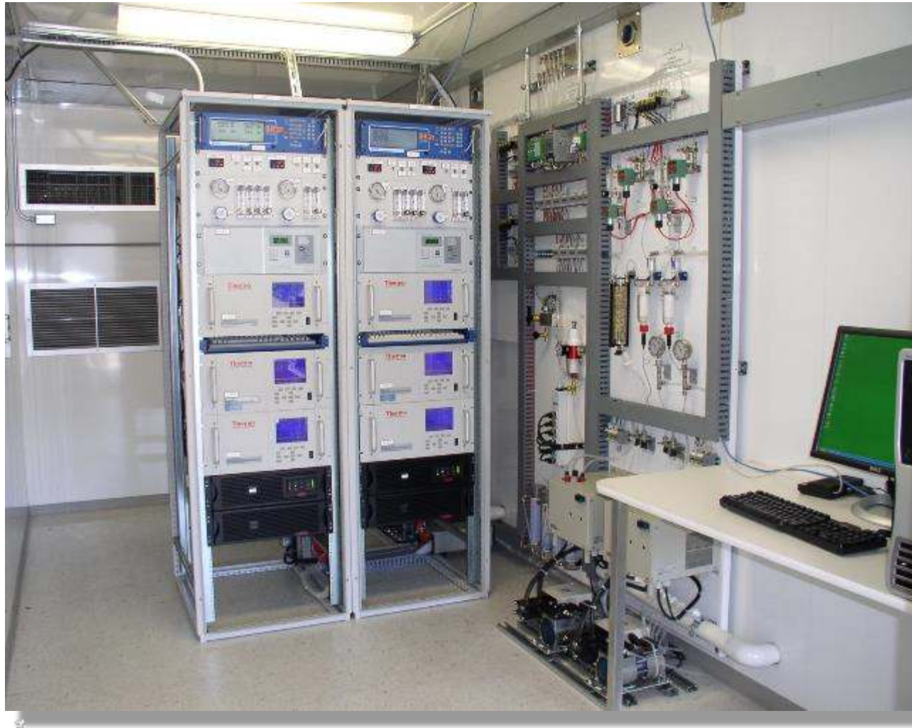
Two Fully Extractive CEMS in a Shelter on natural gas fired turbines with an ESC DAHS measuring NO x , CO and O 2
