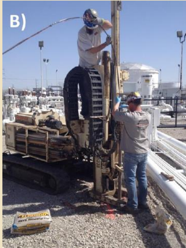
Installation of stick using direct push rig.
